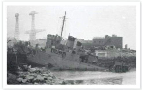
Above: HMS Campbeltown after it ploughed into the dock. The fuses didn't detonate until the next day, but the Germans couldn't haul the behemoth off the gate
